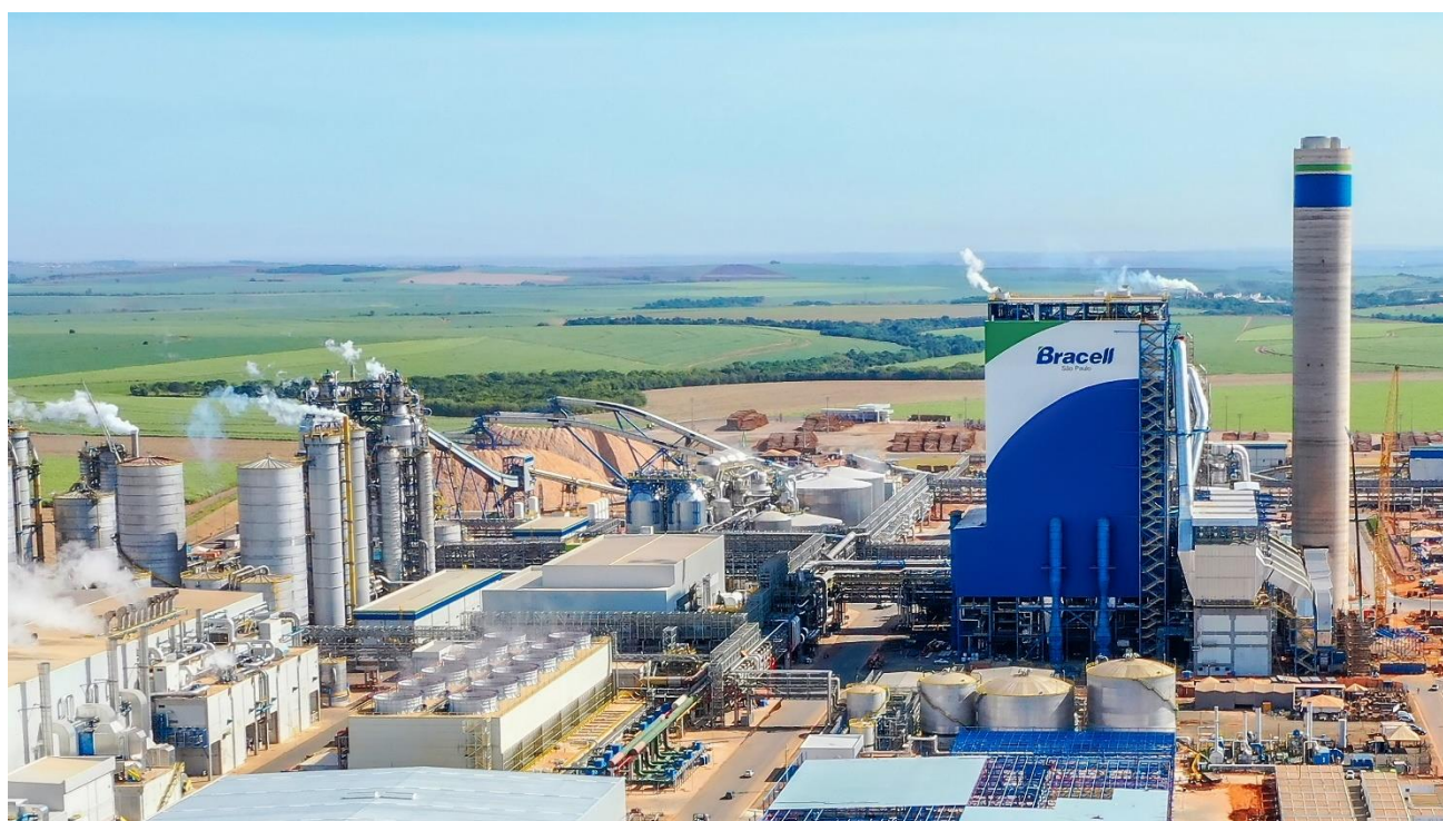
Photo caption: The world’s largest and greenest pulp mill emits steam, not smoke.
